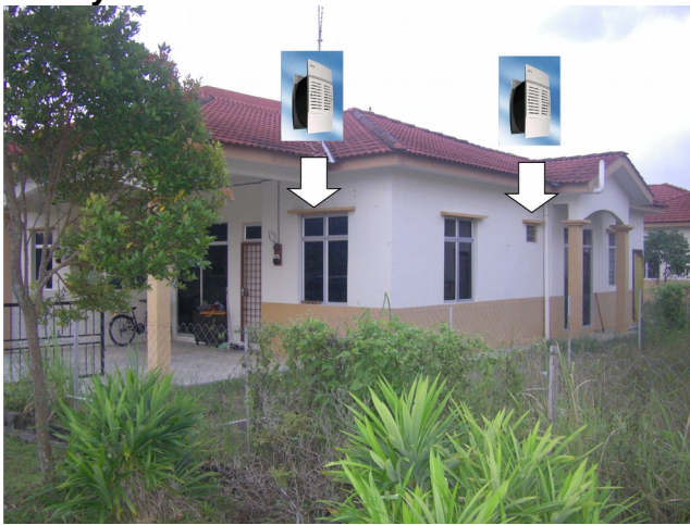
Figure 6: Location of Outside-Ventilators
